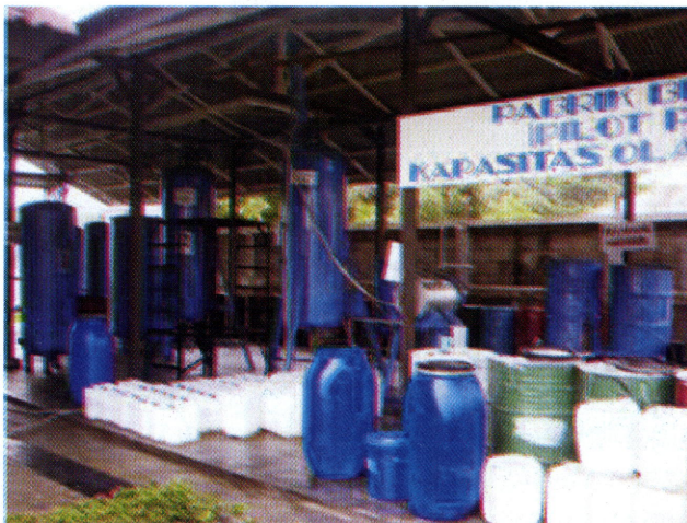
Pabrik Biodiesel Pilot Plant Pusat Penelitian Kelapa Sawit Medan
